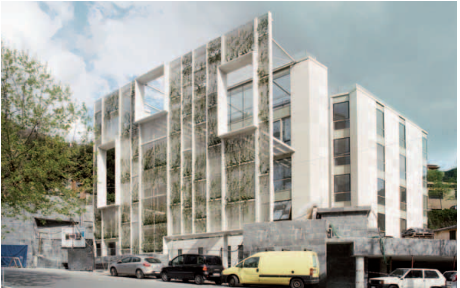
SEA ARTS HOTEL CAMOGLI - IMPERIA (Italy) Design: Studio Gosplan Expanded metal cladding: DELTASYSTEM INTERNATIONAL Photo: © Anna Positano
