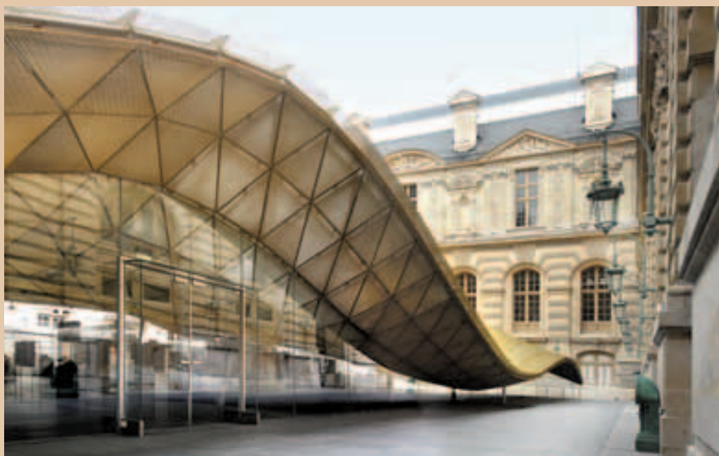
This fluctuating, undulating semi-transparent surface was developed to permit the complementary coexistence of distinctive forms of Islamic art with the Museum's classical 18th century ambience.
