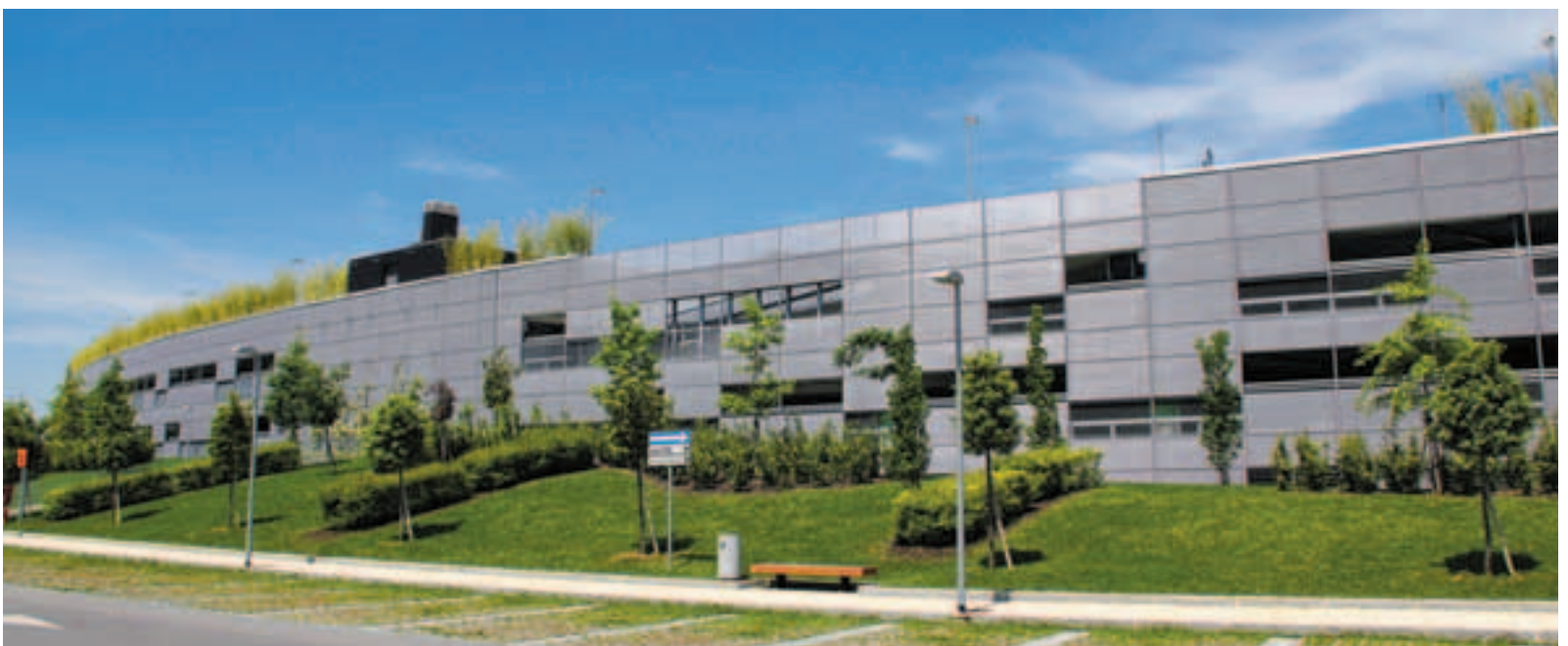
Facing in expanded mesh ensures the passage of air required for multi-storey parking facilities and visually lightens the impact of the not inconsiderable volume with transparency.
